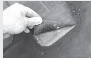
The Bennett roof, which is 20 years old, has reached its end of life. Leaks are patched when discovered, but more extensive long-term solutions would protect the building from costly water damage.
