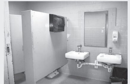
Many bathrooms at the MS/HS have doors that are too narrow to accommodate wheelchairs, and sinks that do not comply with ADA standards.
